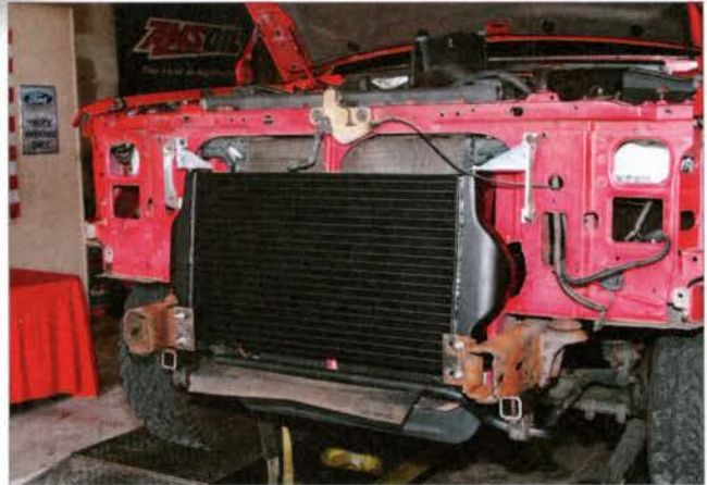
Next on the list was installing the Techni-Cooler.
