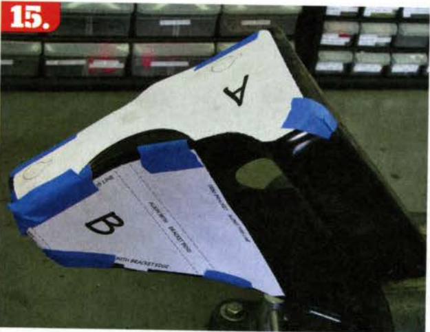
15. To allow room for the Super Scoop to reach the airbox, one of the factory GM braces needs to be modified a bit. Banks supplies fullsize templates in the instructions to ensure installers don't have to figure it out on their own. The cuts still allow the brace to properly function with minimal degradation to its strength.
